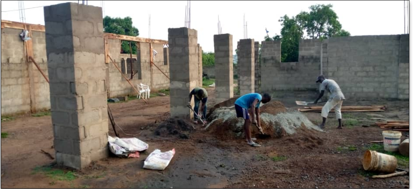
Top picture: Mixing concrete
