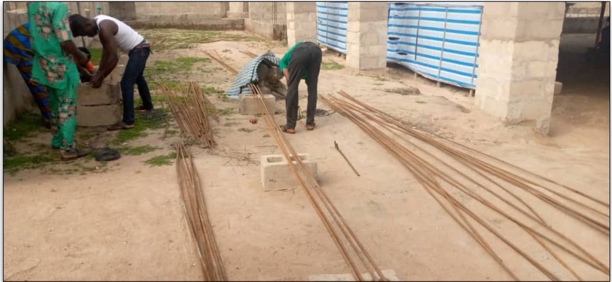
Rebar for reinforcing columns.
