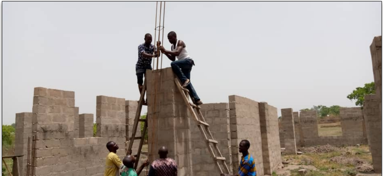
Rebar for reinforcing columns.
