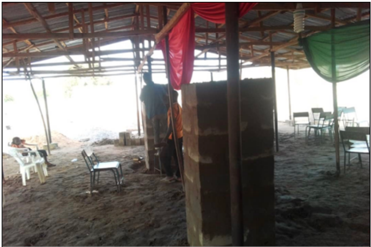
BUILDING THE COLUMNS INSIDE THE CHURCH WITH THE 6 INCH BLOCKS
