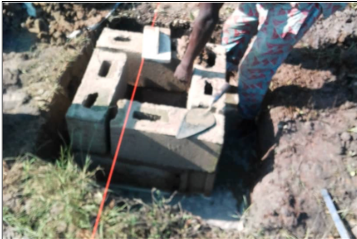
THE MAKING OF THE COLUMNS.
